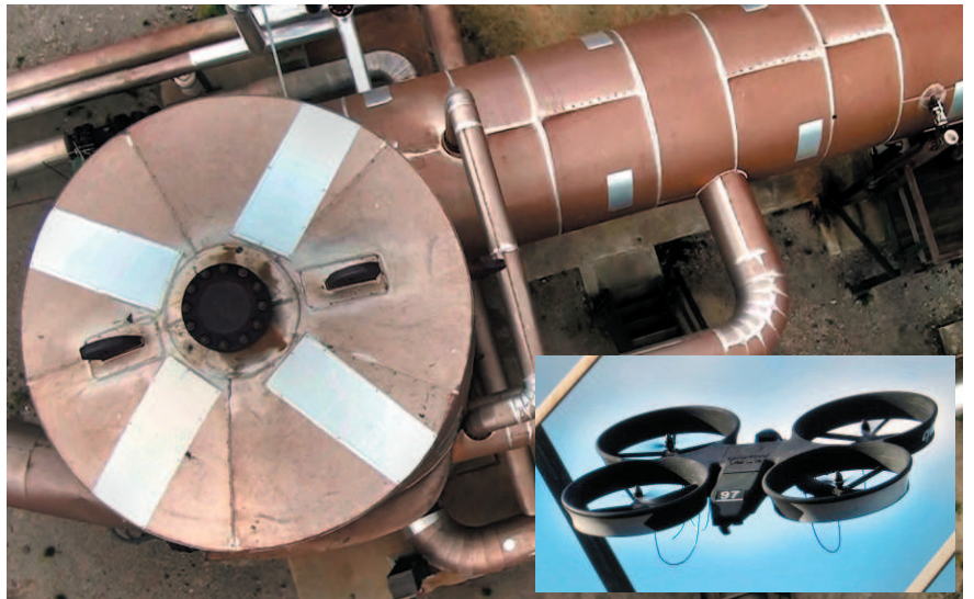
Bioreactor by HERA member PFS Engineering for Contact Energy. This is a plant focused on removing H 2 S from the water discharged from Wairakei PowerStation before it goes into the Waikato river
