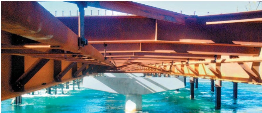
Waitaki Replacement bridge - HERA member Eastbridge supplied 92m and 206m bridges for the upgrade project in the south island. These bridges are weathering steel ladder deck designs and Eastbridge is assisting with the site erection
