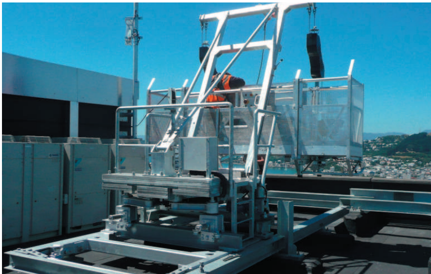
Building Maintenance Unit (BMU) designed by HERA member ETS Engineers designed and installed on Rankine Brown Building of Victoria University, Wellington. The BMU travels around corners with "swing arms" and pivoting bogies.
