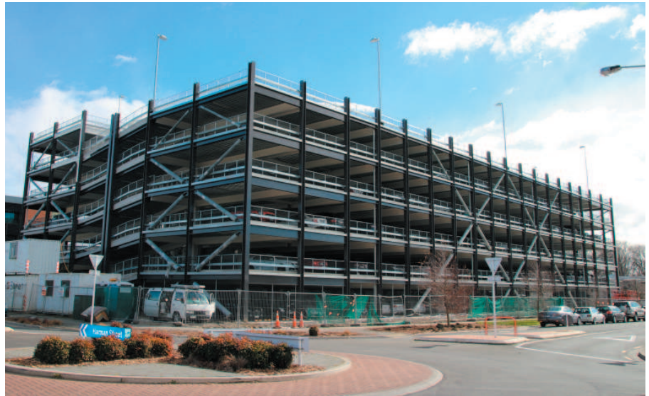
New 5-level car park servicing Christchurch's Hazledean Business Park - a development by Calder Stewart. The steel was fabricated and erected by HERA member Chapman Engineering with the primary floor beams (440 tonnes) supplied by HERA member Steltech Structural
