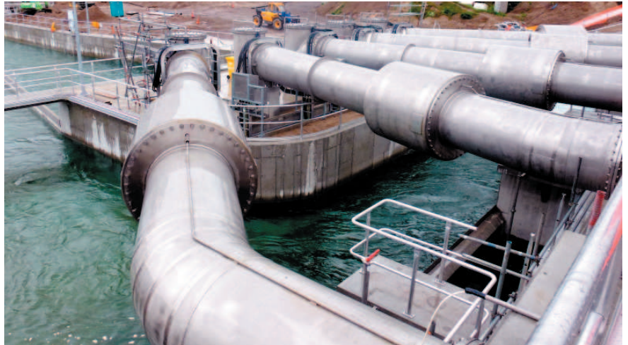
Bioreactor by HERA member PFS Engineering for Contact Energy. This is a plant focused on removing H 2 S from the water discharged from Wairakei PowerStation before it goes into the Waikato river
