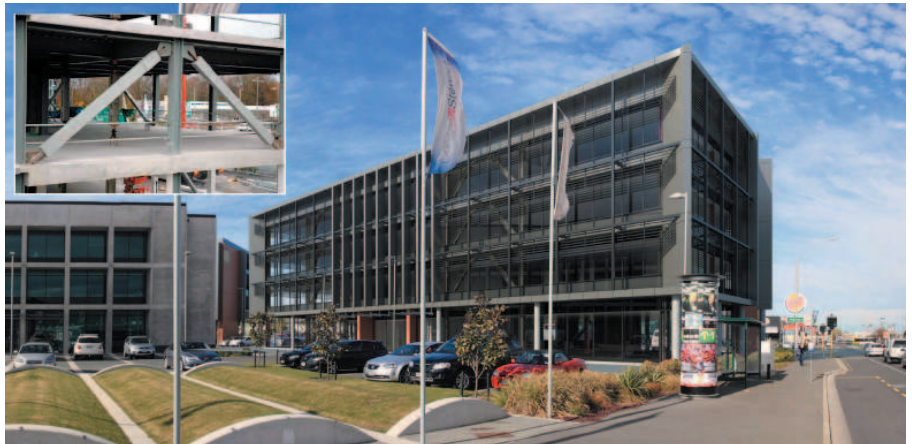
The new 4-level office block in Christchurch's Hazeldean Business Park by Calder Stewart Industries. It incorporates Buckling-Restrained Braces (BRBs) with removable active links recommended by project consultant and HERA member Structure Design Ltd
