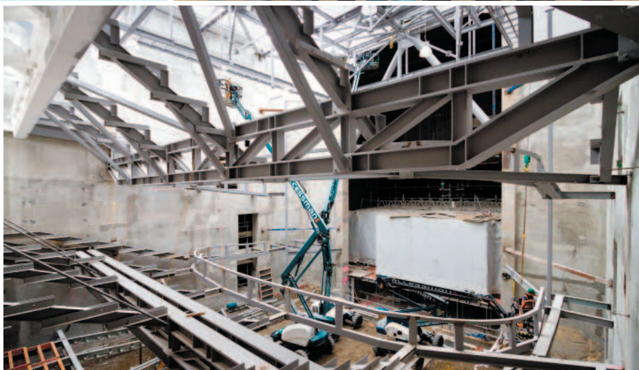
Main structure of the Isaac Theatre Royal in Christchurch fabricated by HERA member Pegasus Engineering. The original building was badly damaged after the earthquake and rebuilt, with strengthening of the original front facade and new roof structure installed
