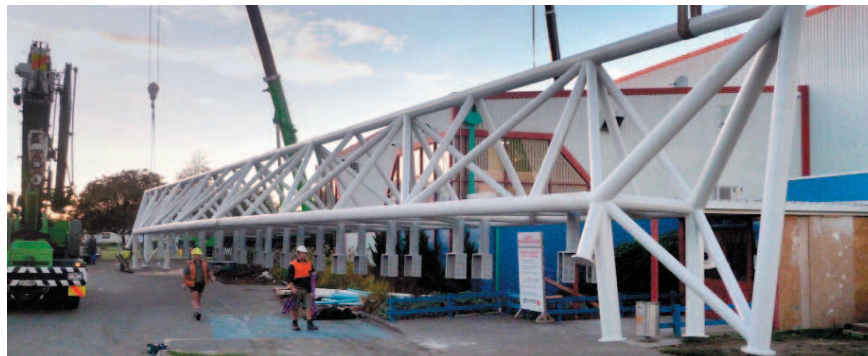
This 45m long 20-tonne seismic strengthening truss for the Flaxmere Waterworld Aquatic Centre was fabricated and painted by HERA member Patton Engineering in their Hastings factory. The truss was transported in one piece.
