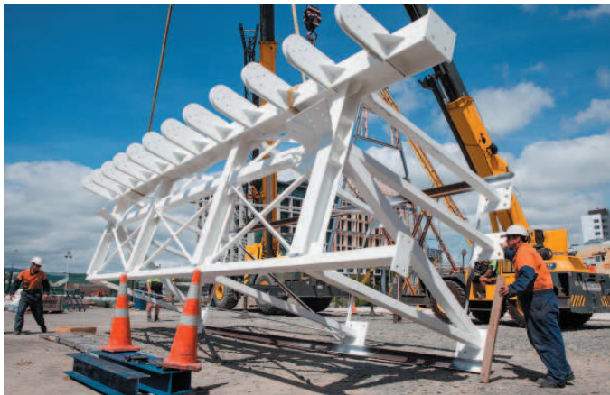
Work on the support structure for the Christchurch cardboard transitional Cathedral by HERA member East Coast Steelwork with design support from HERA member Holmes Consulting Group. While steelwork came in at only 58 tonnes, the structure still stands at 25m tall and holds 700 people
