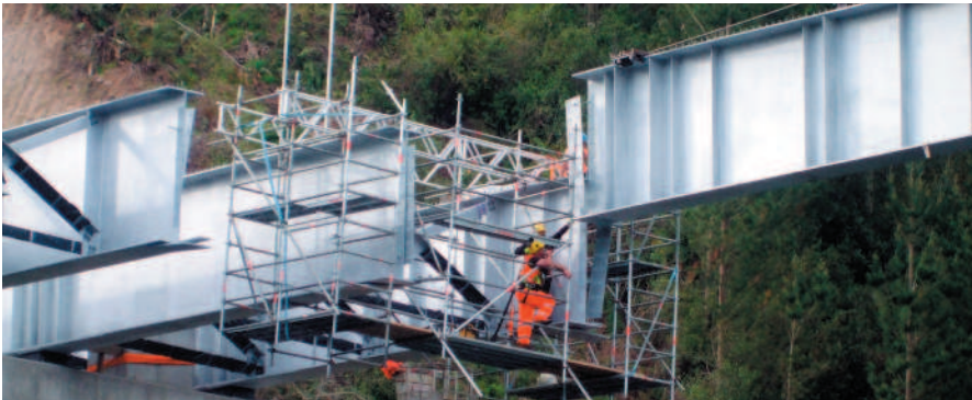
HERA member HEB Structures installing the tandem central beam for the Atiamuri bridge in Taupo. Fabricator and designer are HERA members Grayson Engineering and Bloxam Burnett & Oliver respectively
