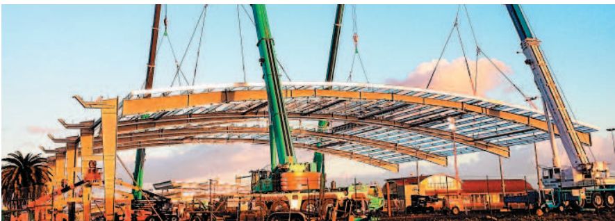
Erection of steel roof for the Bruce Pulman Park Netball Courts, fabricated by HERA member GGE. Total job ended up about 520 tonnes once completed.
