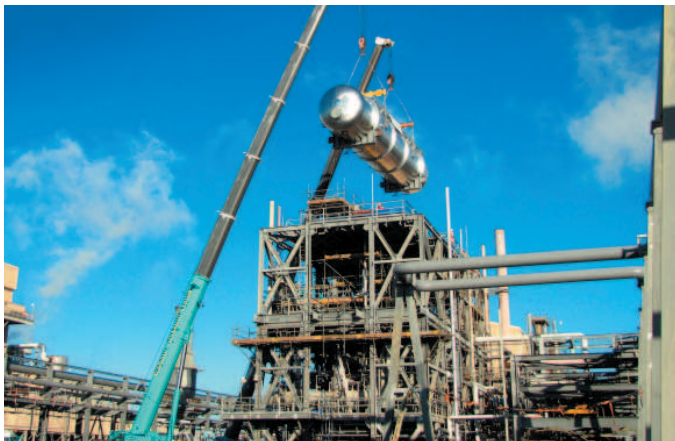
Deaerator vessel fabricated by HERA member Fitzroy Engineering and seen here being installed at the Methanex Motonui plant
