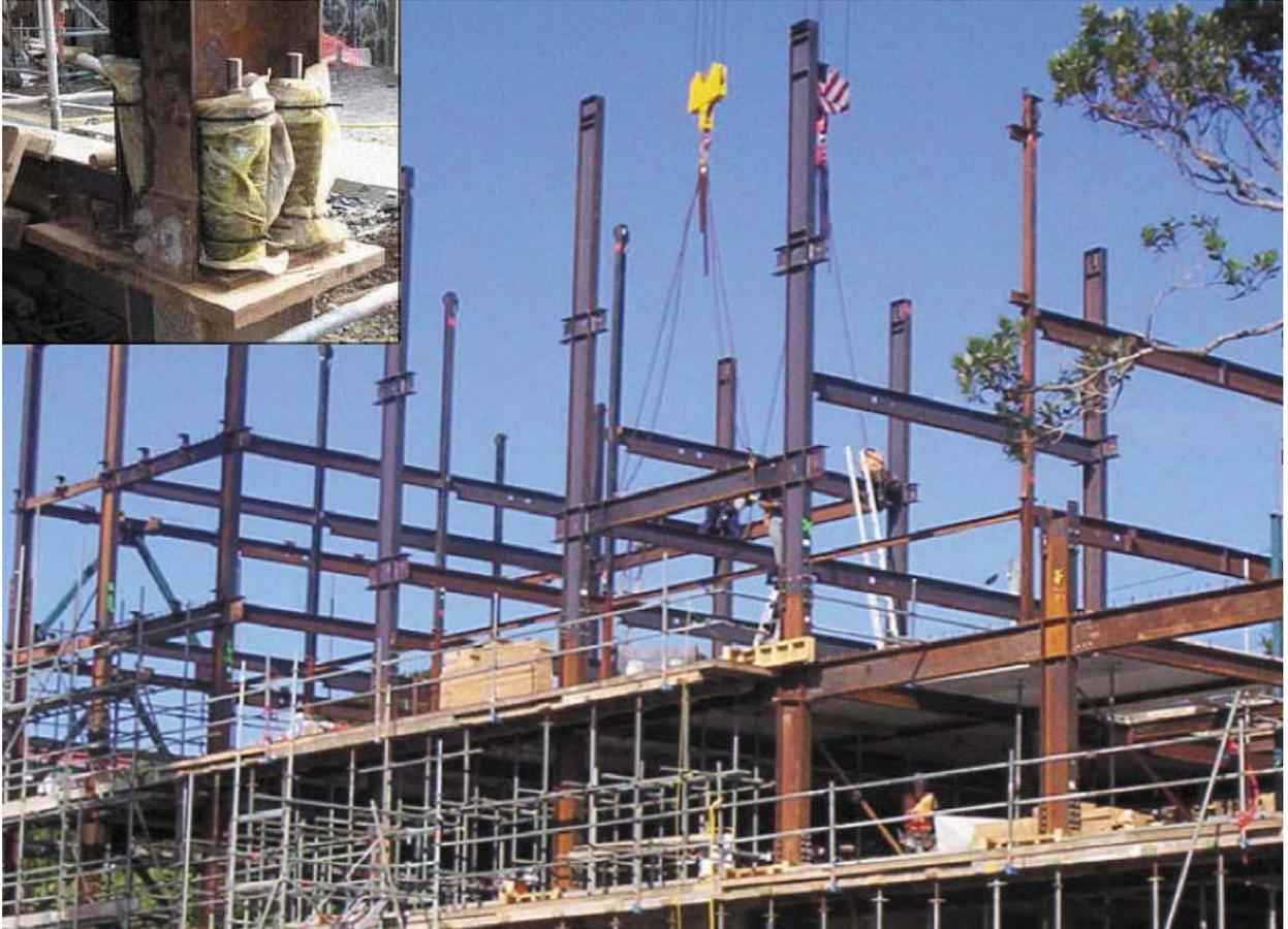
**Figure 7 Aurecon’s International Structural Engineers UK award winning Te Puni student accommodation project which incorporates damage-avoidance rocking frames (inset) and sliding hinges – both developed via Heavy engineering industry levy funded research and government funding.**
